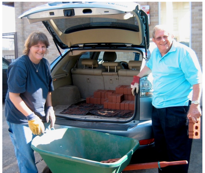
11/4/07 Linda Berard and Vic Appel unloading bricks for the sidewalk in the new patio
